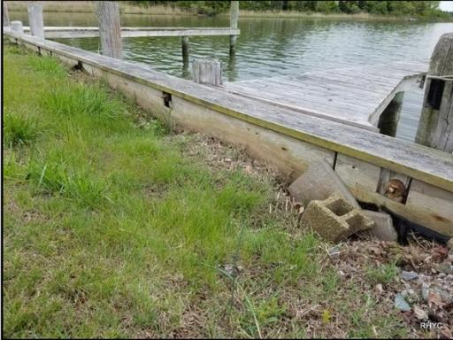
*Figure 4. NE Section of Bulkhead - Spring 2016 - showing one area of washout*
