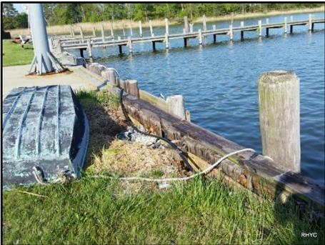
*Figure 5. SW section of bulkhead - Spring 2016 - showing shore washout and deteriorating timber and hardware*
