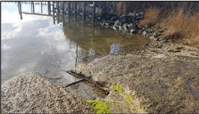
Figure 3. Boat Ramp showing deterioration and exposed rebar
